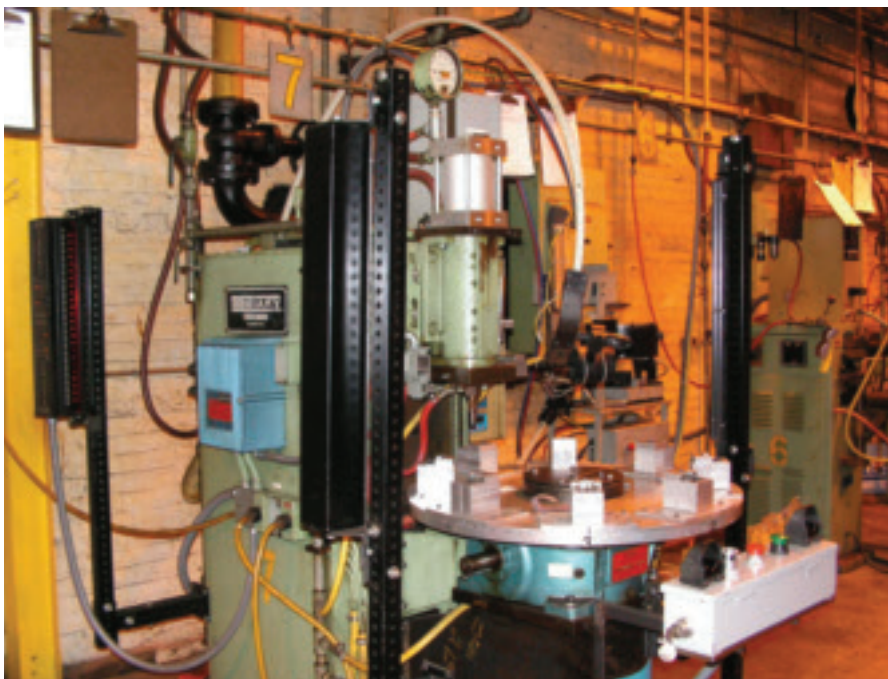
Fig. 5 — Light curtain guarding on all sides protects the operator on this hand-loaded semi-automatic dial table welding machine.
